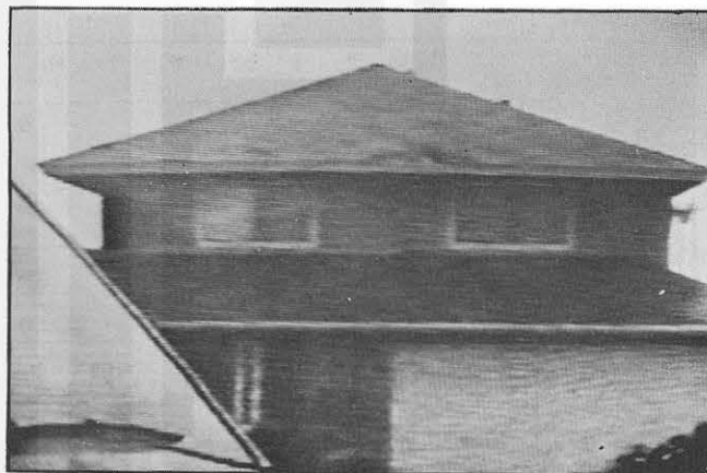
At 173.9 sec, wind diminished and the roof settled down to the 4" (10 cm) bulge.
