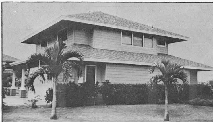
View of the restored house looking west. Southerly winds impinged upon the left-side blew off the roof toward the right.
