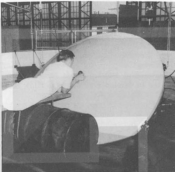
FIGURE 21-2.—Gemini spacecraft during water stability testing.
