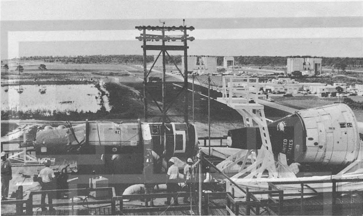
FIGURE 23-1.—Spacecraft and Gemini Agena target vehicle undergoing tests at radar range.
