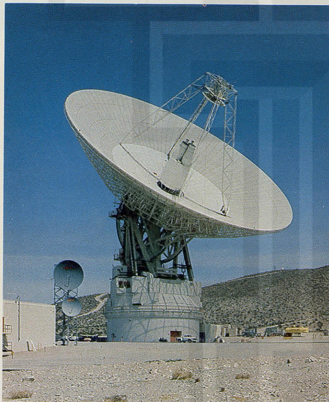
The giant antennae of the world-wide Deep Space Network such as the 64-meter dish at Goldstone, California, will receive the spacecraft radio signals and route them on to Mission Operations for analysis.
