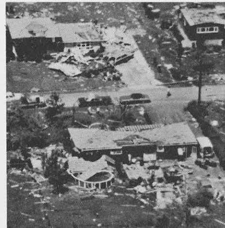
[F1] MODERATE DAMAGE (73 - 112 mph) Peel surface off roofs; mobile homes pushed off foundations or overturned; outbuildings demolished; moving autos pushed off the roads; trees snapped or broken.
