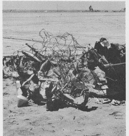
[F4] DEVASTATING DAMAGE (207 - 260 mph) Well-constructed houses leveled; structures with weak foundations blown off some distance; cars thrown and disintegrated; trees in forest uprooted and carried some distance away.
