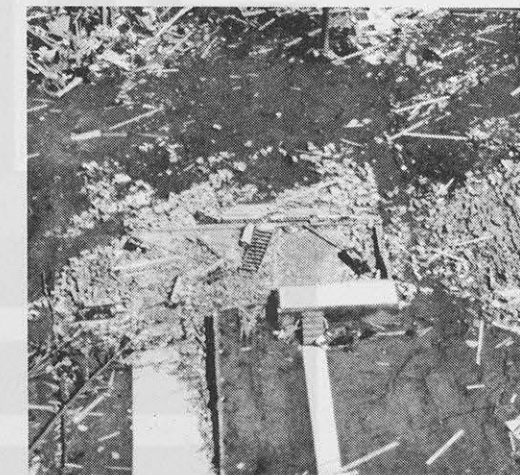
[F5] INCREDIBLE DAMAGE (261 - 318 mph) Strong frame houses lifted off foundations and carried considerable distance to disintegrate; automobile-sized missiles fly through the air in excess of 300 ft; trees debarked; incredible phenomena will occur.
