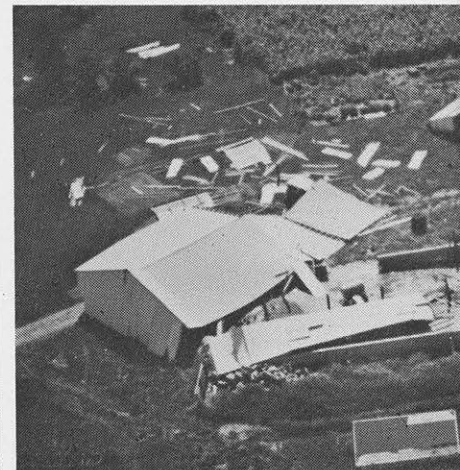
[F1] MODERATE DAMAGE (73 - 112 mph) Peel surface off roofs; mobile homes pushed off foundations or overturned; outbuildings demolished; moving autos pushed off the roads; trees snapped or broken.
