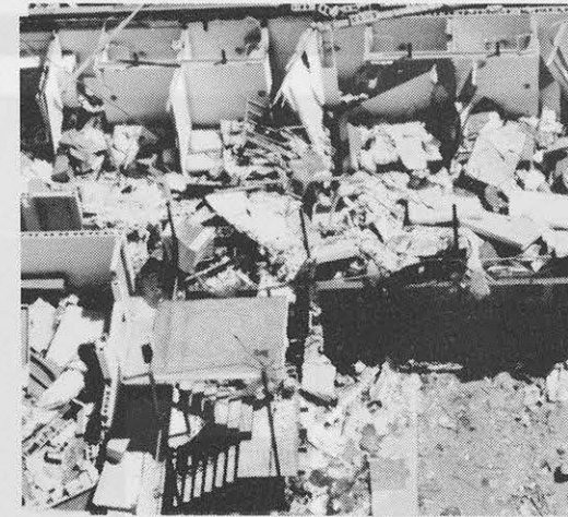
[F3] SEVERE DAMAGE (158 - 206 mph) Roofs and some walls torn off well-constructed houses; trains overturned; most trees in forest uprooted; heavy cars lifted off the ground and thrown; weak pavement blown off the roads.
