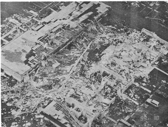
Left: A Naranja Lakes condo oriented in the wind-perpendicular (broadside) direction. The roof was lifted into a vertical position and dropped upside-down after a 180° rotation. Connected and broken tie-beams weighing one ton per 20 ft are visible on the downwind side. Fujita photo 1253 EDT 9/14/92. Right: Mobile homes at Naranja Lake oriented by luck in the wind-parallel (streamline) direction. Fujita photo 0906 EDT 9/8/92.
