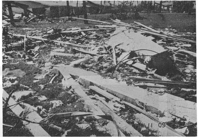
Left: Tie-beams at Pine Woods Villa (see map) blown apart by a mini-swirl. Continental Aerial Survey photo taken on 8/27/92. Right: Ground view of the tie-beams. Fujita photo 1109 EDT 9/9/92.
