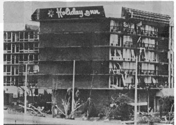
Above: A view of some of the wind damage to NHC's communications equipment atop the IRE Financial Building. The radar dome of the WSR-57 weather radar was blown off the highest structure seen at the center right of the photograph. (Photo courtesy: Roger Edwards) Above(right): The Holiday Inn at Cutler Ridge, north of Homestead, suffered extensive wind damage with nearly every window blown out! (Photo courtesy: NHC) Below(left): Outside wall almost completely removed from the east side of an apartment building in the Saga Bay development, near Cutler Ridge. Below(right): Partial removal of the outside wall from the south (right) and west faces of the building. (Photo courtesy: Roger Edwards)
