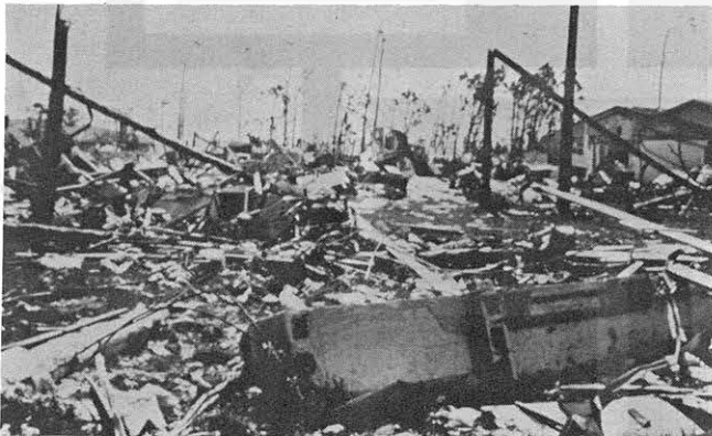
Above(left): Ground view of the devastation in the Pinewoods Villa. In the foreground are broken segments of a large tie beam. Above(right): Another ground level view in the Pinewoods Villa. (Photo courtesy: NHC)
