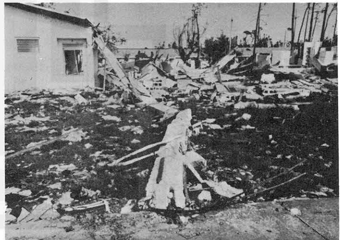
Left: Aerial photo of a tie-beam (see map) blown off toward the west. Fujita photo 1245 EDT 9/14/92. Right: Ground view of the tie-beam reinforced with one-inch steel rods. Fujita photo 1649 EDT 9/15/92.
