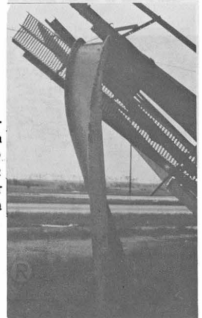
Right: An 18-inch wide structural I-beam bent and twisted in the Naranja community. (Photo courtesy: Ralph Clark) Left: Another royal palm tree near Homestead was pierced by a wind driven sheet of plywood. (Photo courtesy: NHC)
