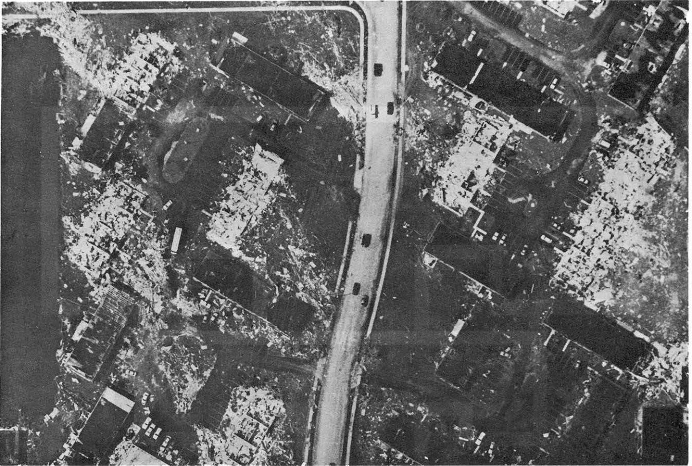
Center of Andrew's eye passed directly over Naranja Lakes, resulting in a 180° shift of the first wind from NNW into the second wind from SSE. Many buildings oriented WSW-ENE (wind-perpendicular) direction received the f3 damage while those in the NNW-SSE (wind-parallel) direction were spared. Enlargement of a Continental Aerial Survey photo taken on 8/26/92.
