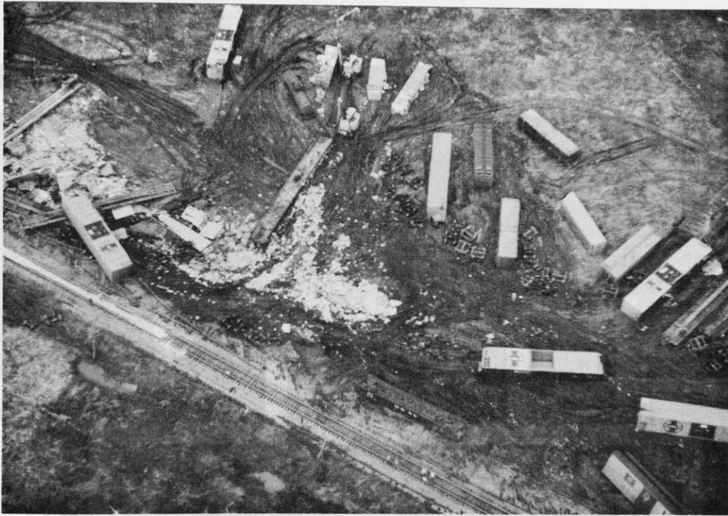
Fig. 10. A close-up areal view of Santa Fe freight cars. Since the derailment blocked the trunk line connecting Chicago with Kansas City, repair crew started working during the night.
